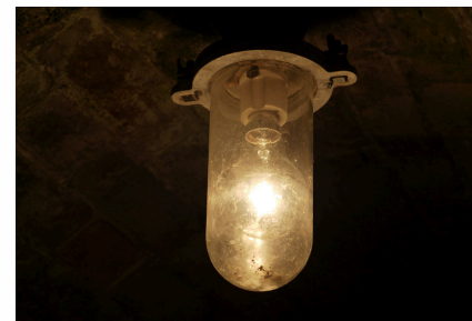
A1: Existing bell jar luminaire
